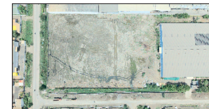
▲ Shakti Drip Plant
