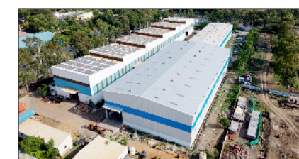
▲ Shakti Energy Solution GI line Plant
